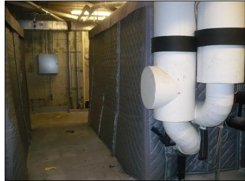
HUSH FLEX™ Enclosure with Cutouts for Water Pipes
