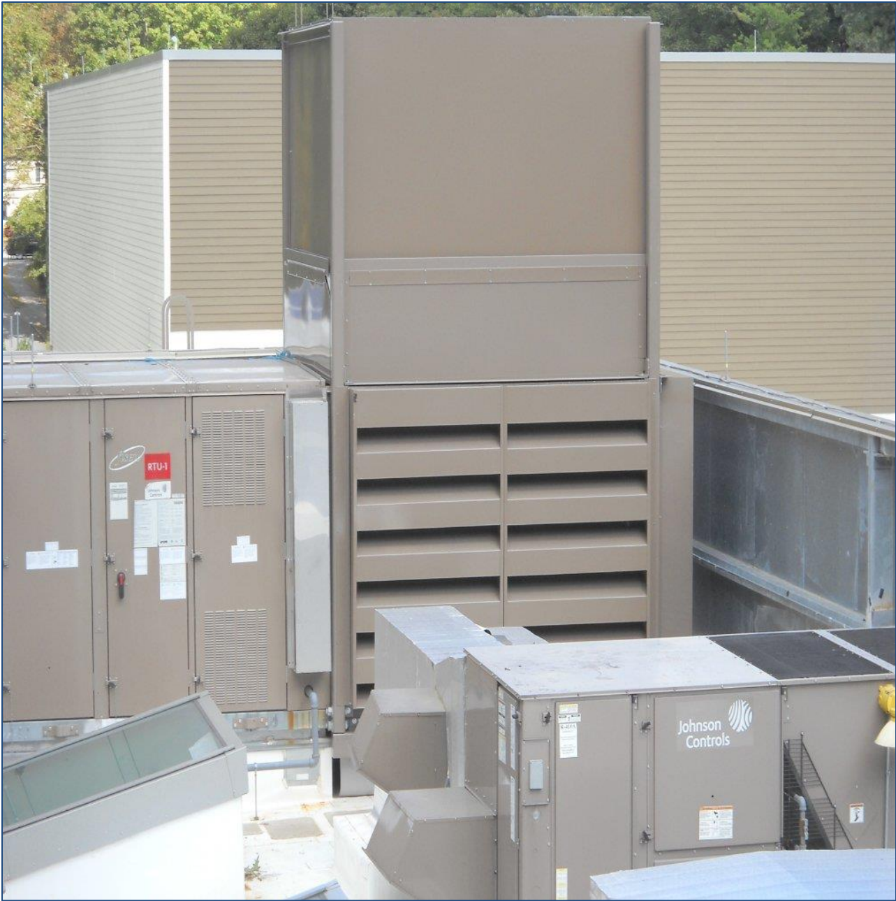
Condenser Section Enclosure
