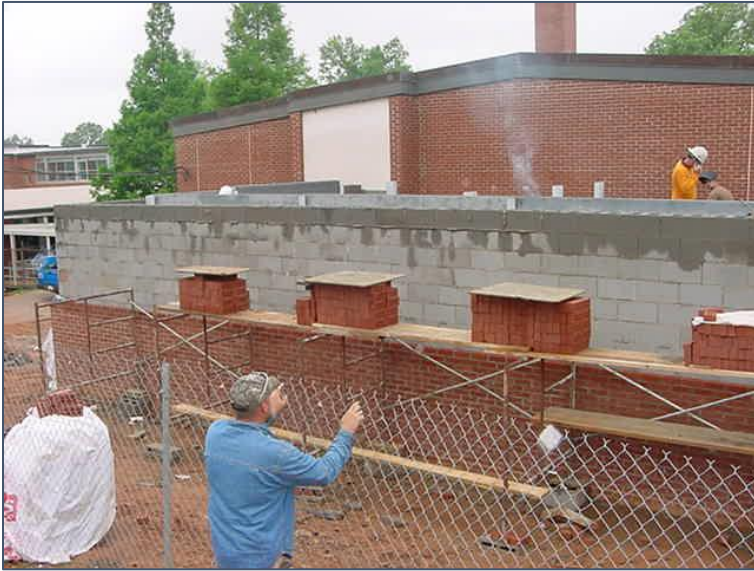
Installation of Brick Façade to Match School Building
